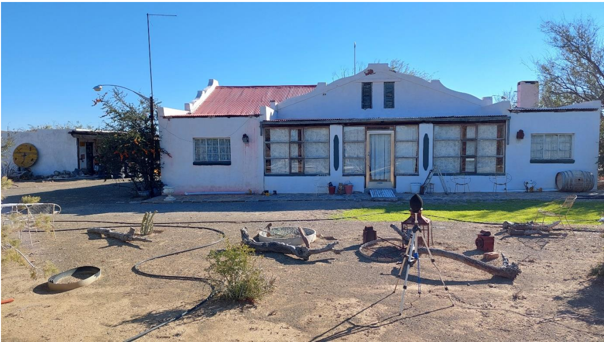
Photos B.1: Measurement location at SGEKLTSL01
