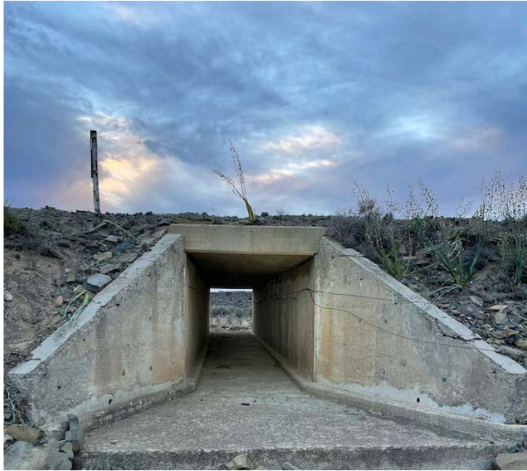
Figure 15: Culverts which could provide roosting opportunities
