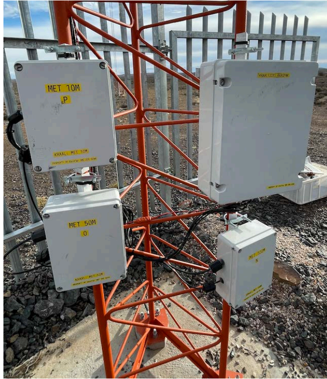
Figure 2: Bat monitoring equipment on the met mast
