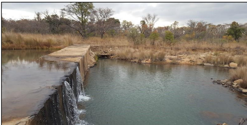
Plate 8 Site photo taken in a North Western direction
