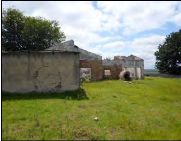
Figure 32. Structures at KP 21.
