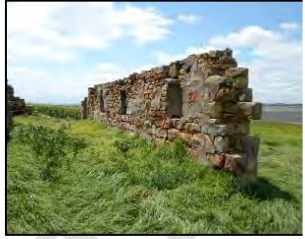
Figure 37. Wall at KP 22.
