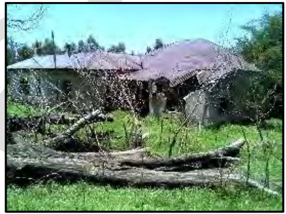
Figure 22. General site conditions.
