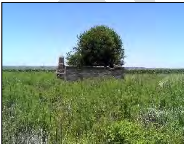
Figure 17. Structure at KP6.
