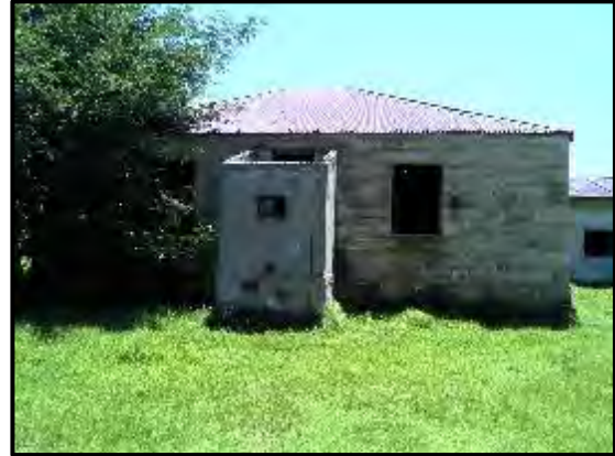
Figure 20. Structure with hipped roof.
