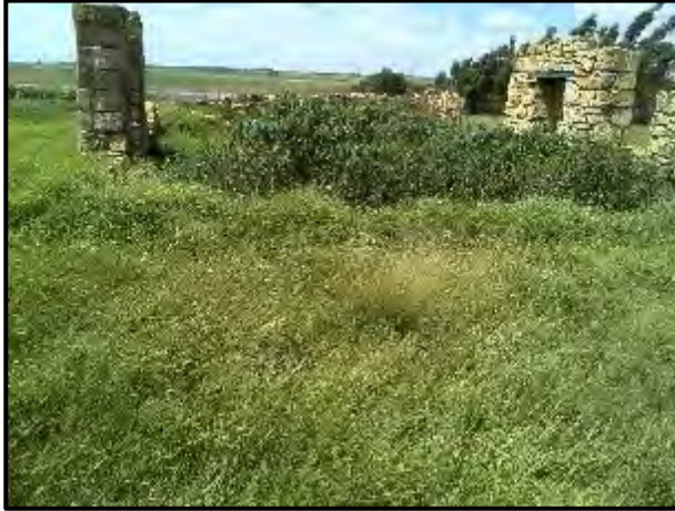
Figure 24. Sandstone structure at KP 12.
