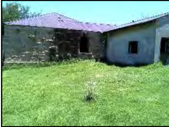
Figure 19. Structure with added on plastered sections.
