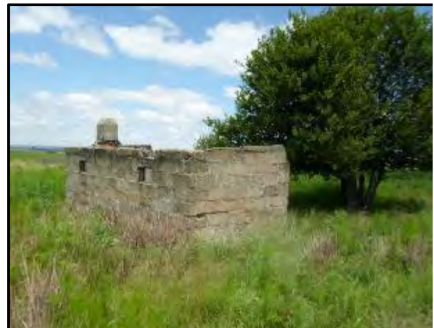
Figure 18. Structure at KP 6.
