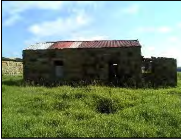
Figure 30. Outlying buildings still in use.
