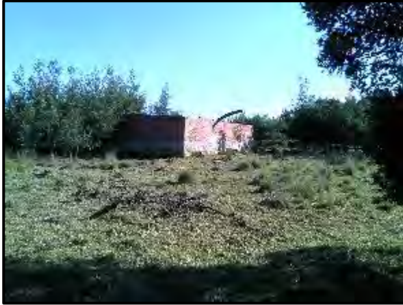
Figure 23. Structure at KP 11.
