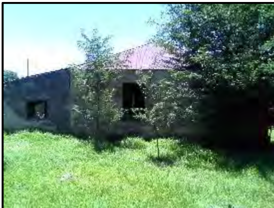
Figure 21. All the fittings have been removed.
