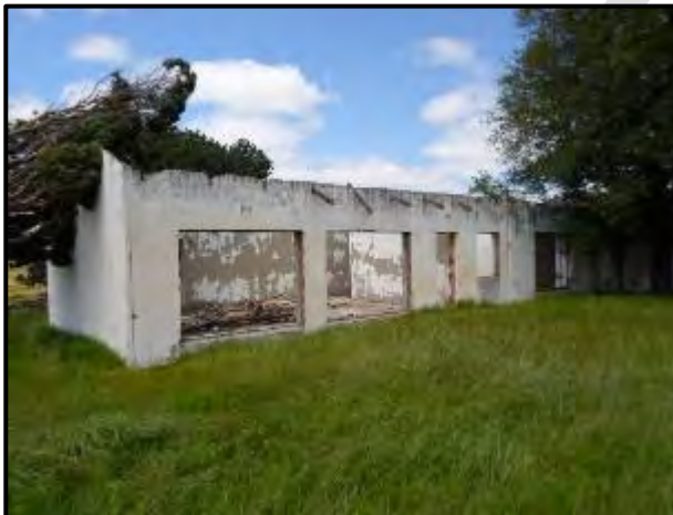
Figure 34. Structures at KP 21.
