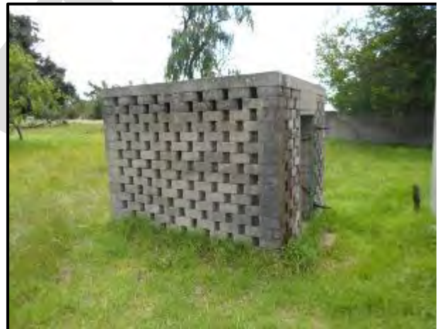
Figure 35. Structures at KP 21.
