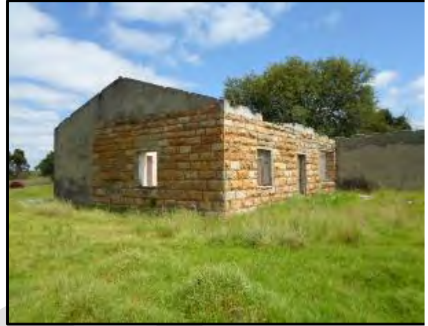
Figure 33. Structures at KP 21.
