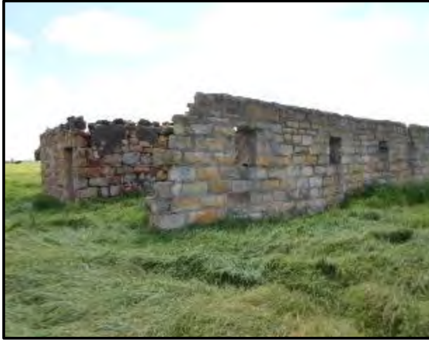
Figure 36. Structure at KP 22.
