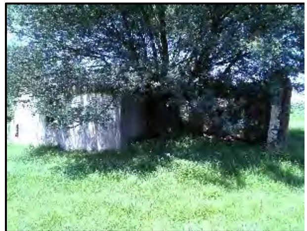
Figure 29. General site conditions at KP 15.
