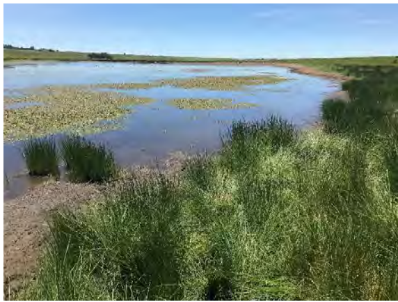
An artificial impoundment constructed within a valley-bottom wetland area, which allows for permanent surface water features to develop.
