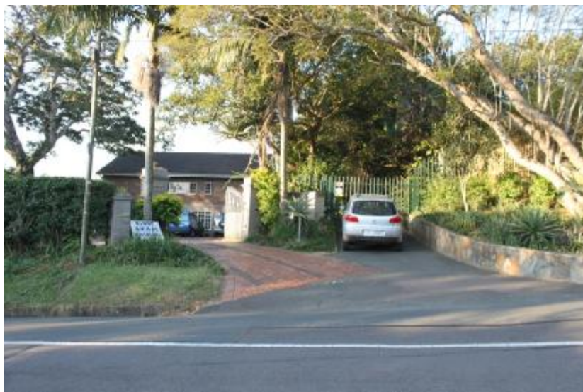
5 Krantzview Road (Erf 5184) & neighbouring property 7 Krantzview Road from Krantzview Road
