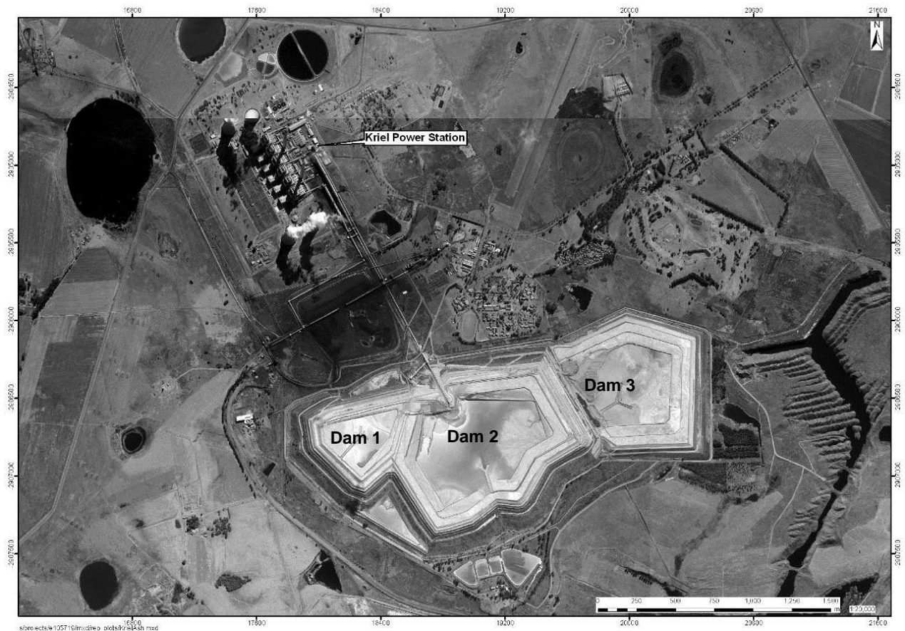
Figure 1-2 | Aerial photograph of the Kriel Power Station and existing ash dam complex
