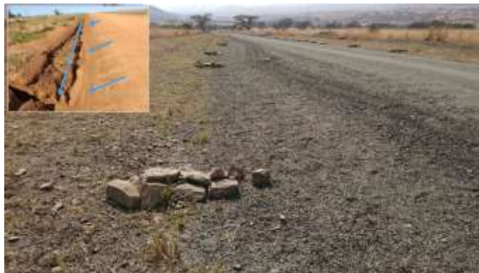
Figure 6-7 Example of road margin erosion prevention
