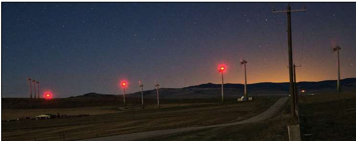
Figure 22: Aircraft warning lights fitted to the wind turbine hubs (Source: http://www.pinchercreekecho.com/2015/04/29/md-of-pincher-creek-takes-on-wind-turbine-lights )
