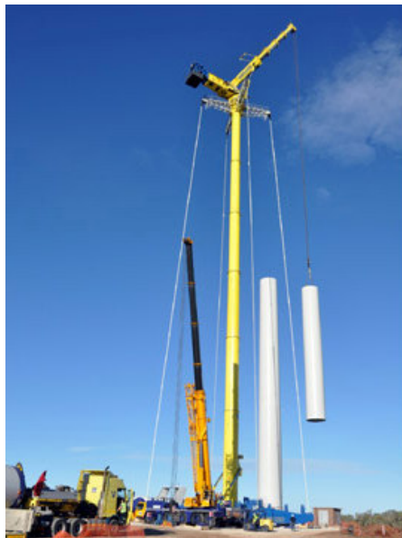
Figure 4-5: Cranes at work
