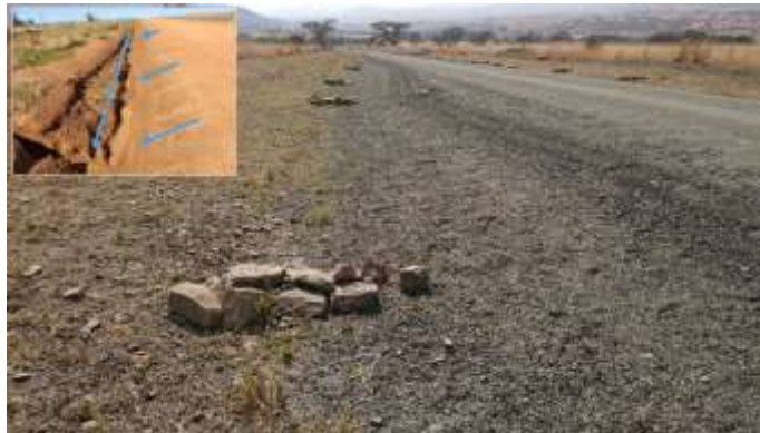
Figure 3-7 Example of road margin erosion prevention
