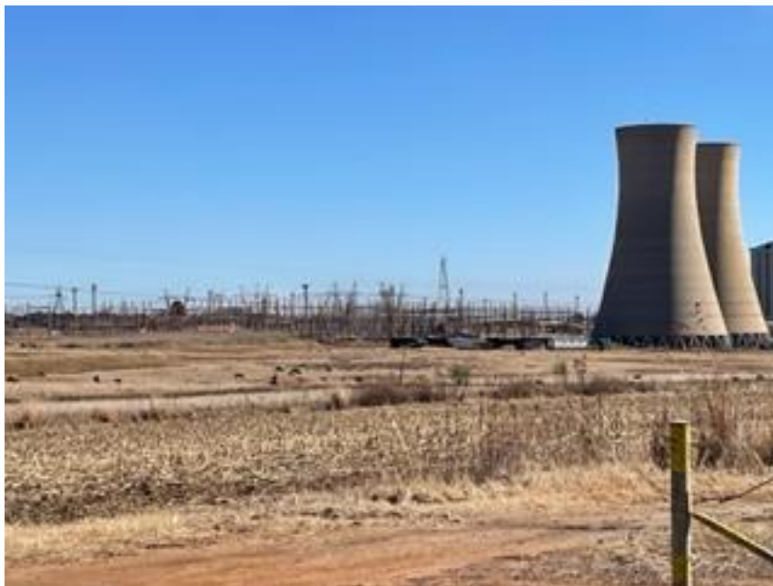
Figure 1: Partial view of Komati Power Station with Kudu Substation to the left
