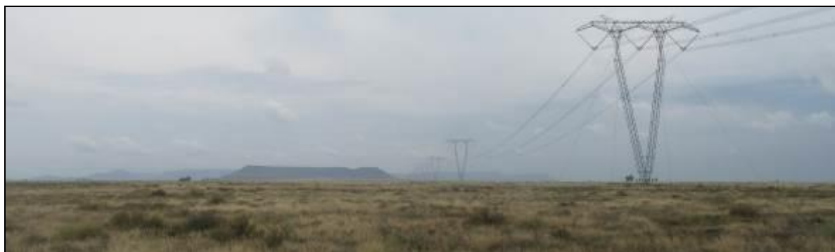
Photograph 3.4: Transmission line crossing the road between Tafelkop and Wolwekuil (42/RE) west of the PV 12 site, Basberg (mountain) in the background
