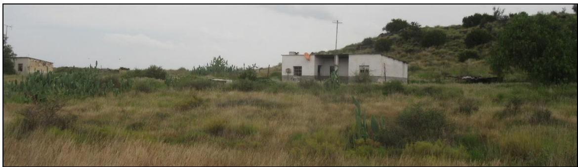
Photograph 3.6: Inhabited labourer's dwelling on Basberg
