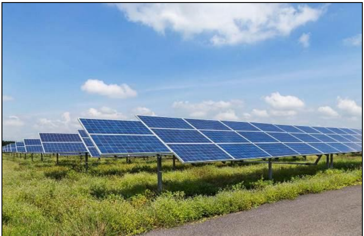
Photograph 1.1: Typical PV SEF facility
