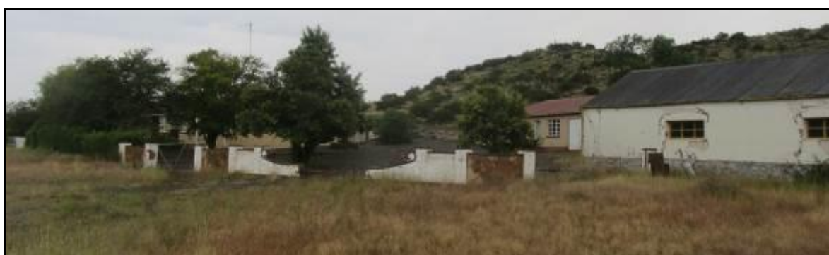
Photograph 3.5: Uninhabited farmstead and outbuildings on Basberg
