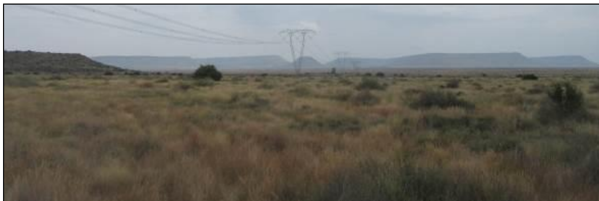
Photograph 3.4: 765 kV line traversing Basberg approximately 500 m west of the farmstead.
