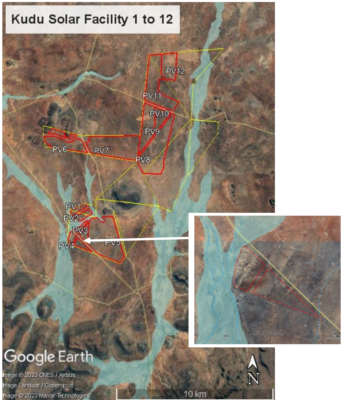
Figure 2. Proposed project elements under consideration in this specialist assessment. Note that the full extent of the land portions (shown in yellow) serves as the study area. This report is focused on Kudu Solar Facility 4 (PV4).
