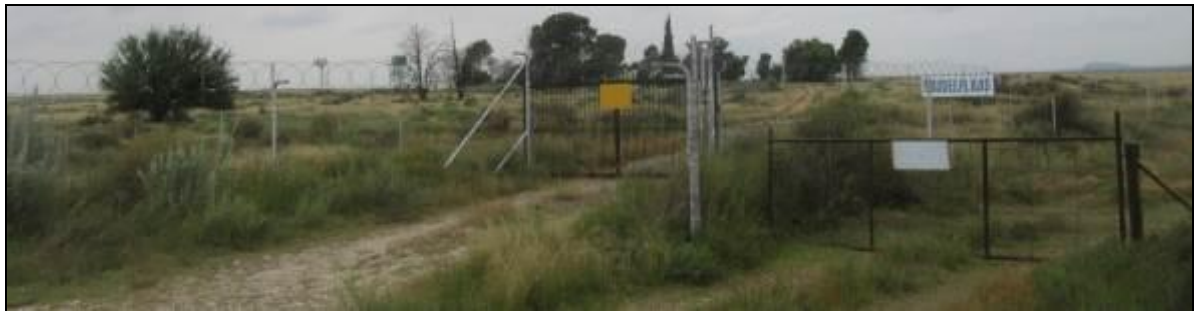
Photograph 3.6: Entrance to Middelplaas.
