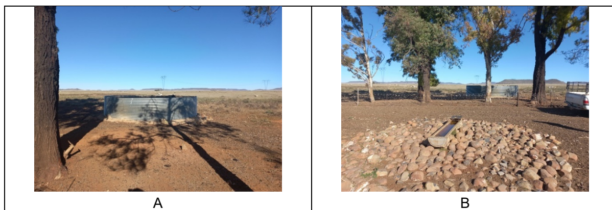
Figure 3-12: A) HBH22 pipeline dam, picture taken in an east-south-easterly direction. B) HBH22 pipeline dam and water trough, picture taken in a south-south-westerly direction. Photos: ABO Wind.
