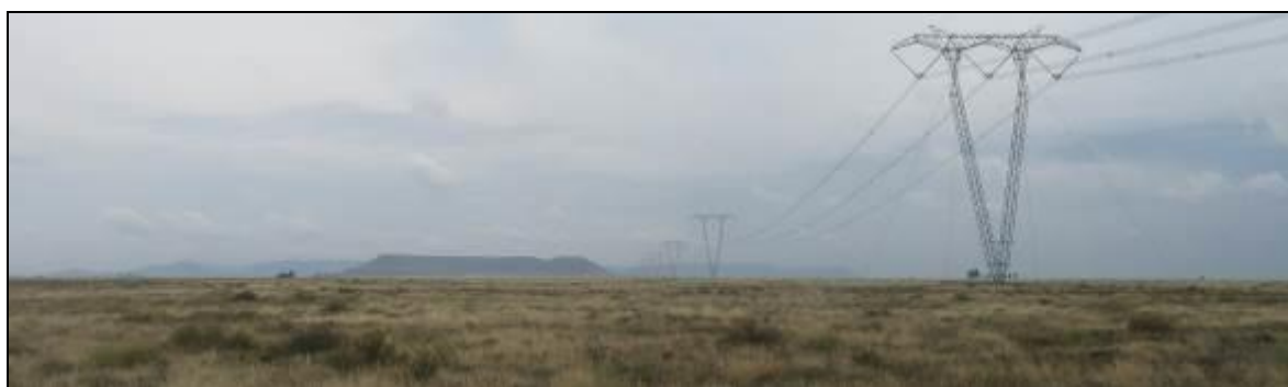
Photograph 3.4: Transmission line crossing the road between Tafelkop and Wolwekuil (42/RE) west of the PV 7 site, Basberg (mountain) in the background
