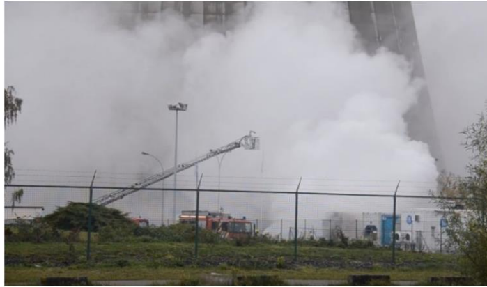
A fire engulfs a lithium-ion battery system at an Engie test site in Belgium, Nov. 11.
