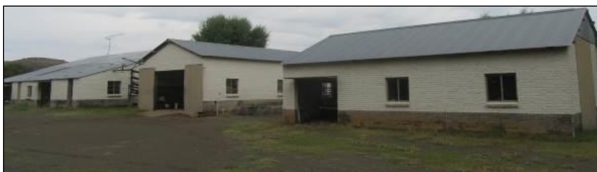
Photograph 3.5: Farm buildings on Wolwekuil yard.
