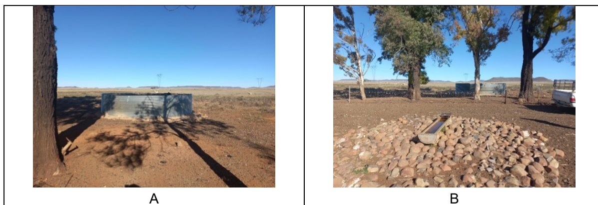
Figure 3.14: A) HBH22 pipeline dam, picture taken in an east-south-easterly direction. B) HBH22 pipeline dam and water trough, picture taken in a south-south-westerly direction. Photos: ABO Wind.
