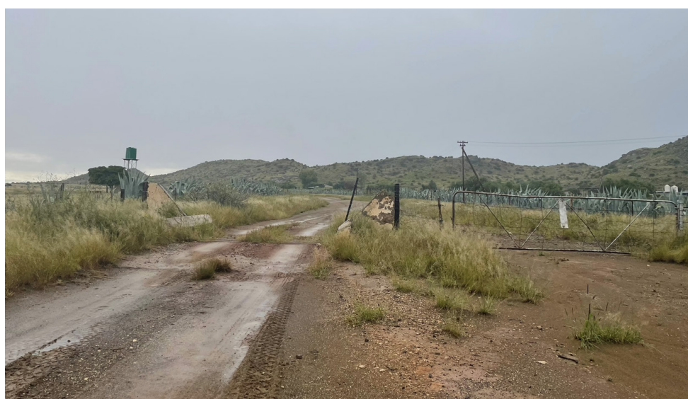
Figure 2.11: Potential Access Route Option 3: Divisional Road 3096 (Photograph taken from the R48) (Sturgeon, 2022)
