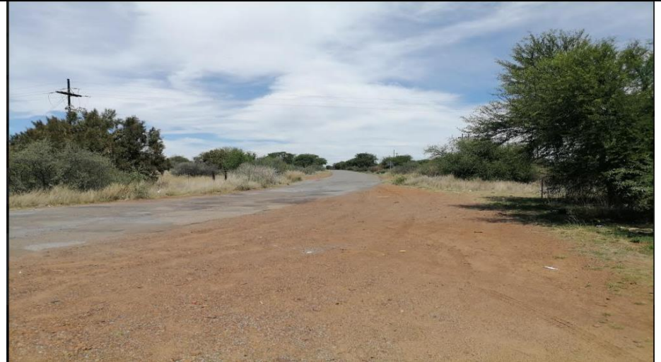
Existing road that will be widened.
