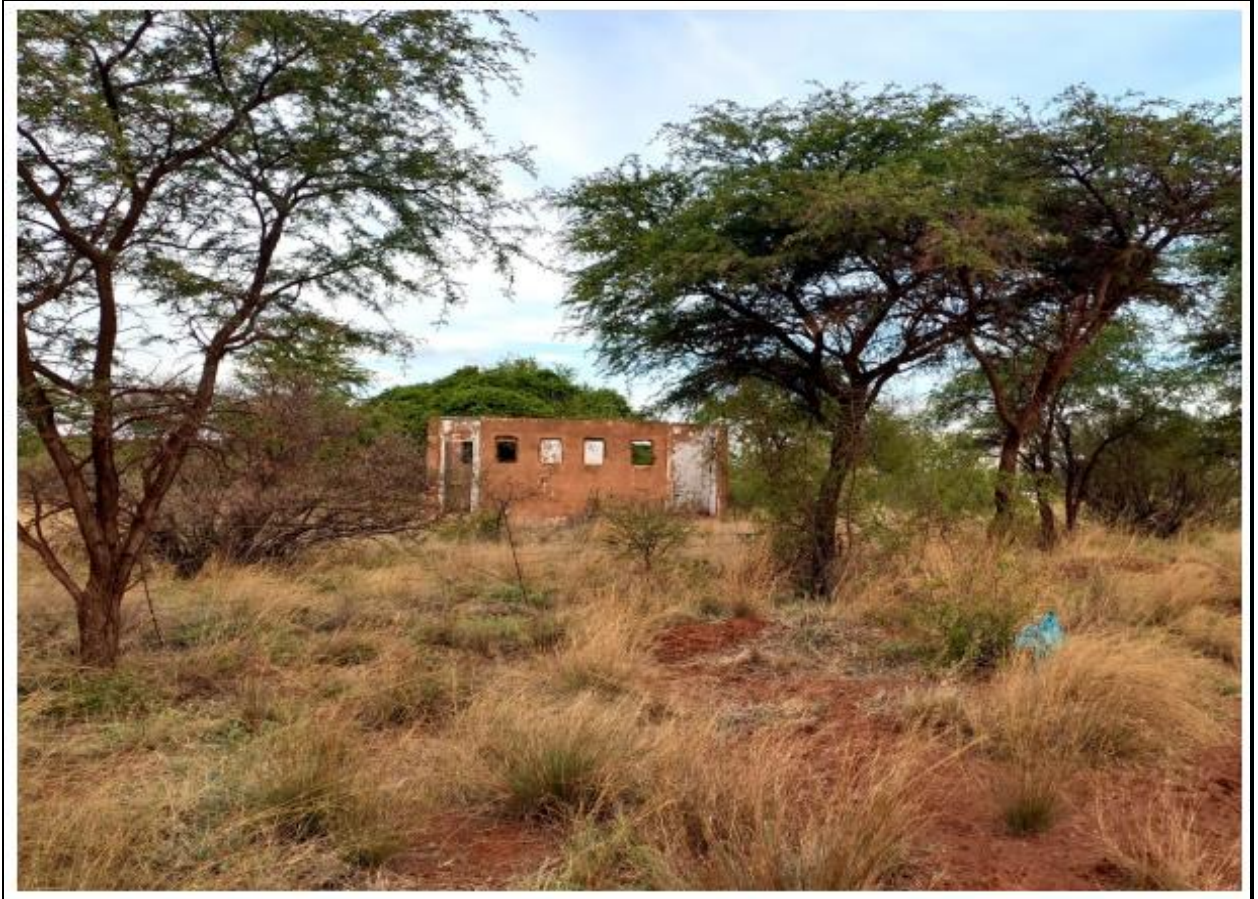
Figure 16: Remnants of buildings
