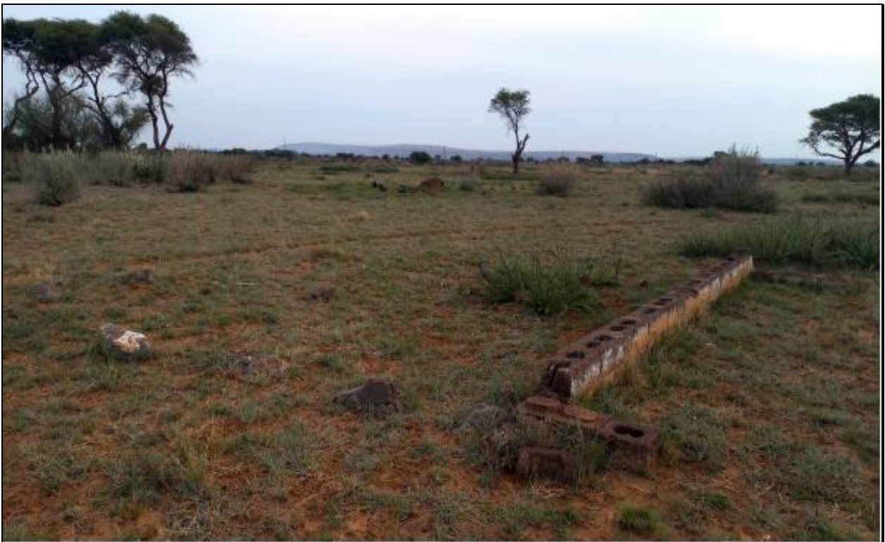
Figure17: Demolished building remains
