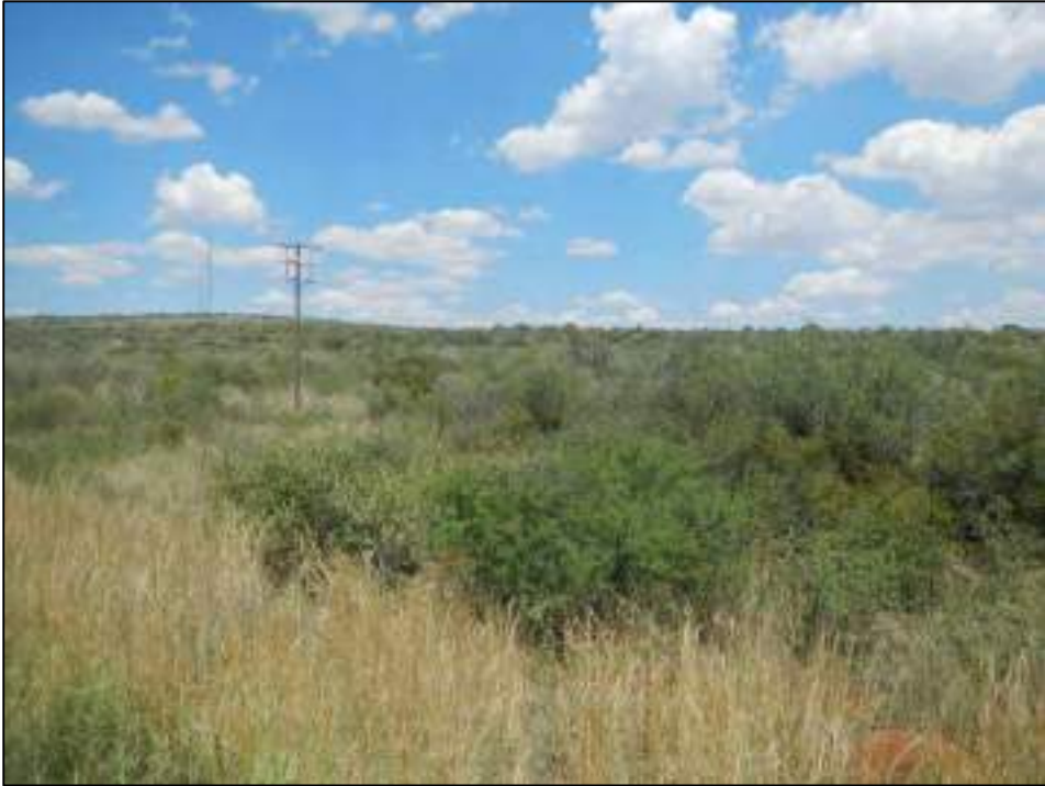
Figure 11: Typical view of the telephone lines which can be found within the study area
