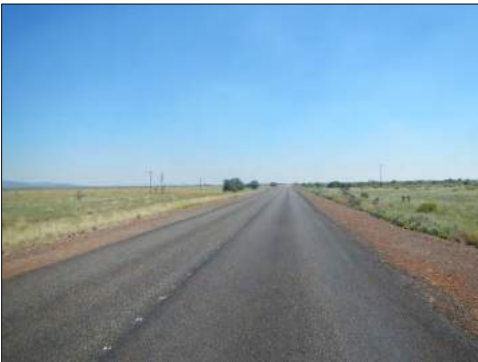
Figure 14: Typical view of the R31 main road
