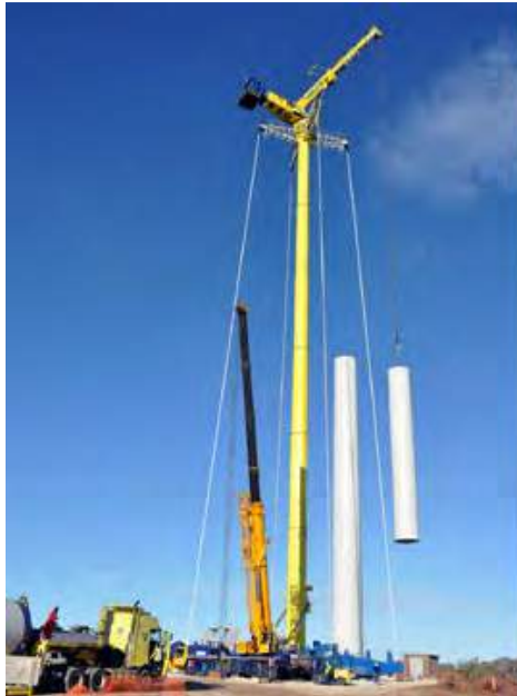
Figure 14: Cranes at work
