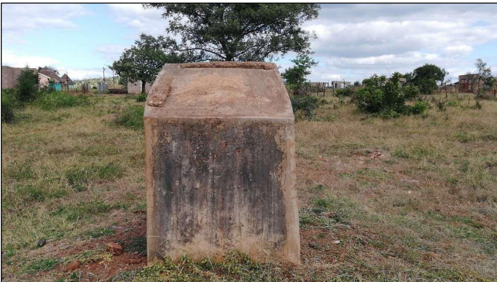
Figure 87: Pedestal of rehabilitated shaft.
