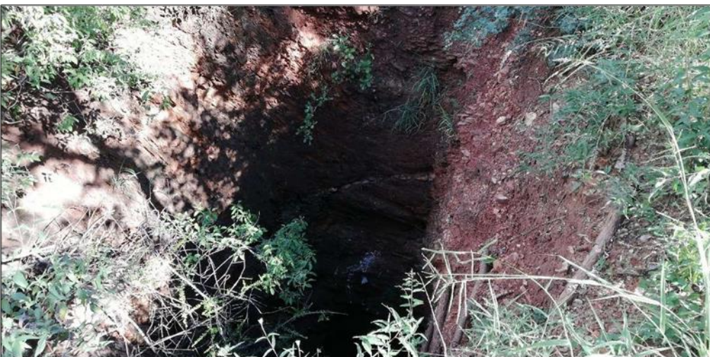
Figure 83: Vertical shaft at proposed Pit 05.
