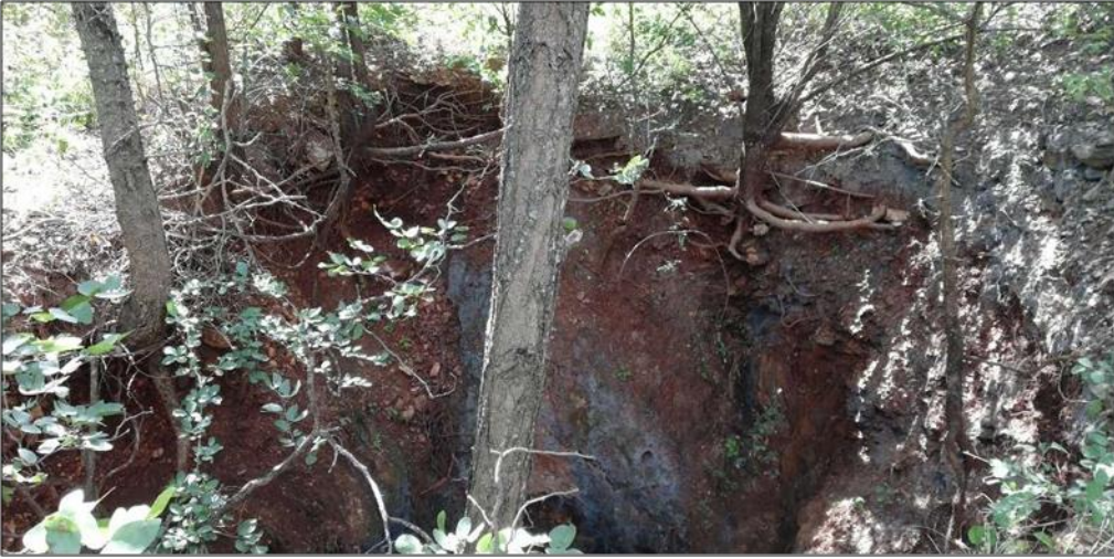
Figure 84: A second vertical shaft at proposed Pit 05.
