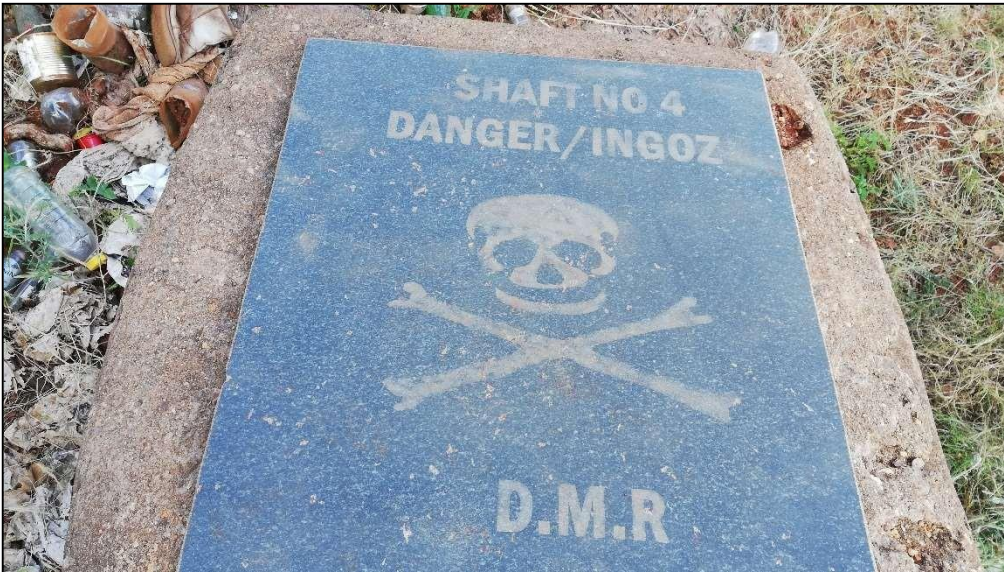
Figure 30: Granite top of rehabilitated shaft No 4.
