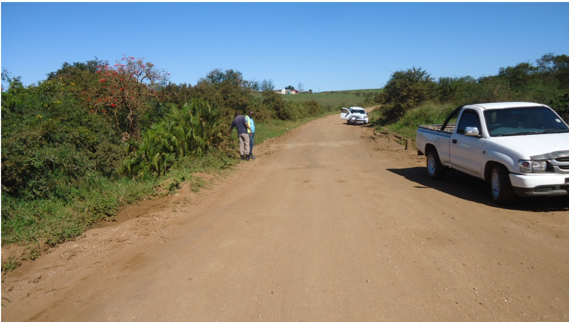
Culvert four - courtesy of Henwood and Nxumalo Consulting Engineers
