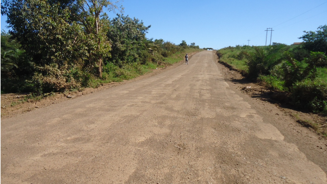
Culvert three - courtesy of Henwood and Nxumalo Consulting Engineers
