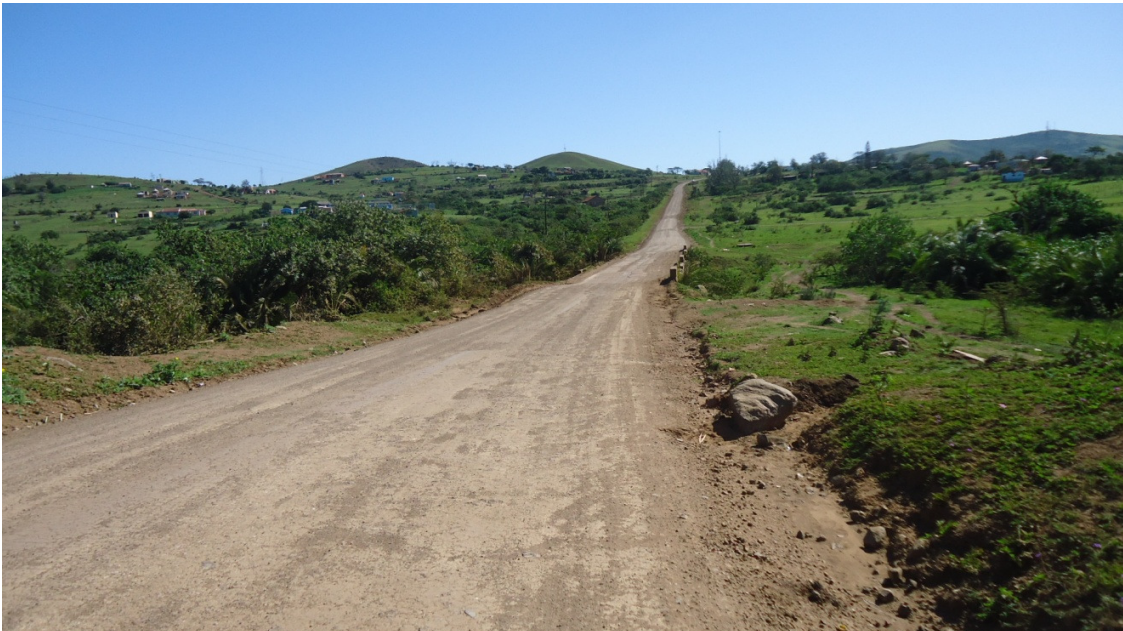
Culvert two - courtesy of Henwood and Nxumalo Consulting Engineers
