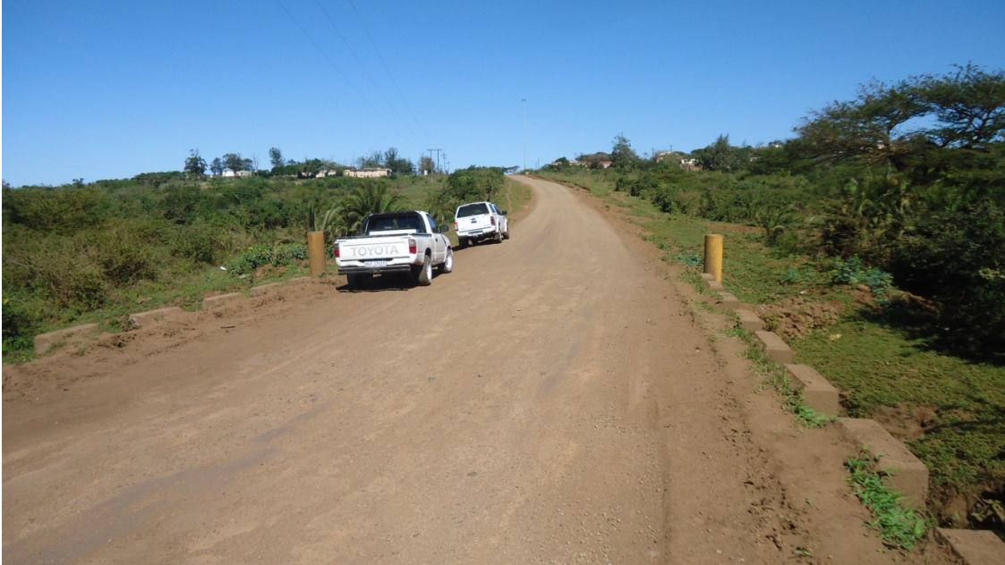
Culvert one - courtesy of Henwood and Nxumalo Consulting Engineers
