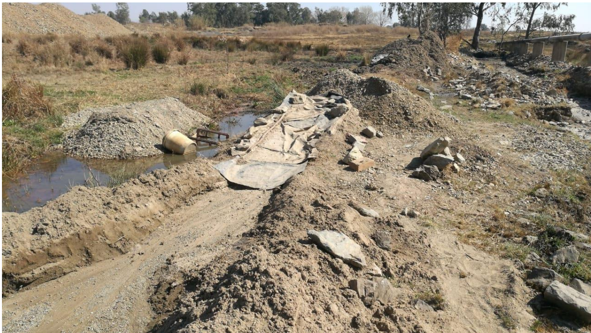
Figure 3: Illegal mining undertaken along the pipeline route
