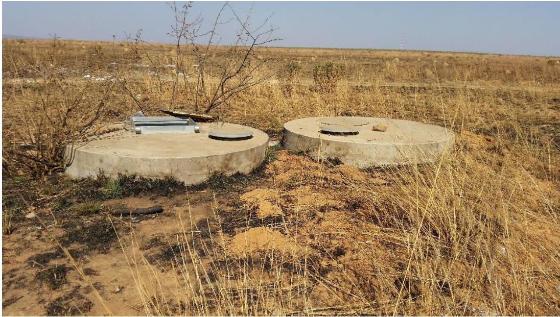
Figure 4.4: Sewer and water pipeline servitude are seen in the surrounding area of the site
