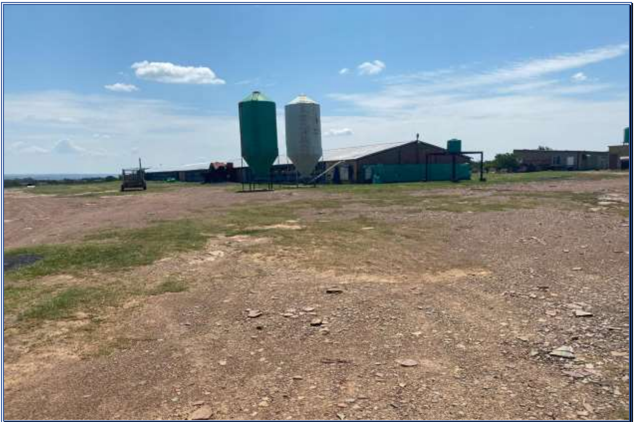
Picture 5: Broiler Unit onsite
