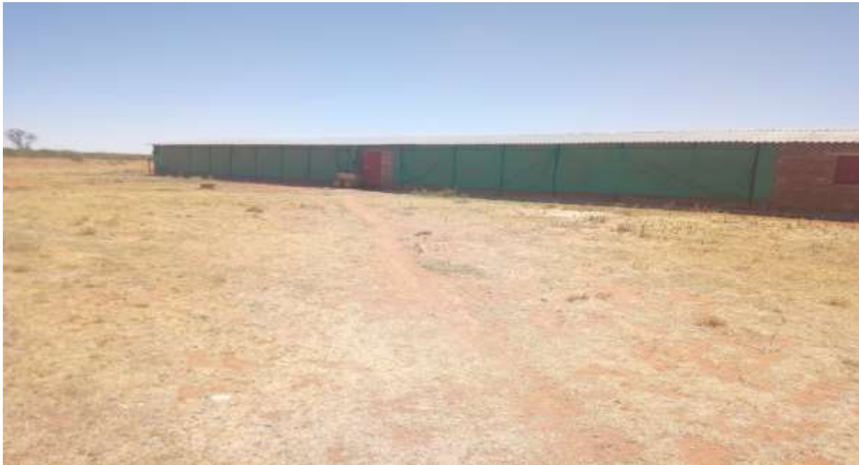
Figure 3: Canvas is rolled up or down to control the temperature inside the house. Mesh ensures that no rodents or birds can enter the house and possibly spread disease.
