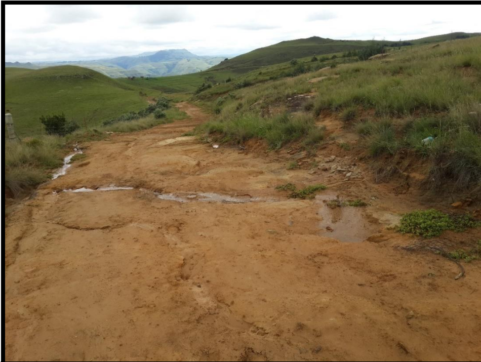
Photo 1: Showing drainage line in relation to the road.
