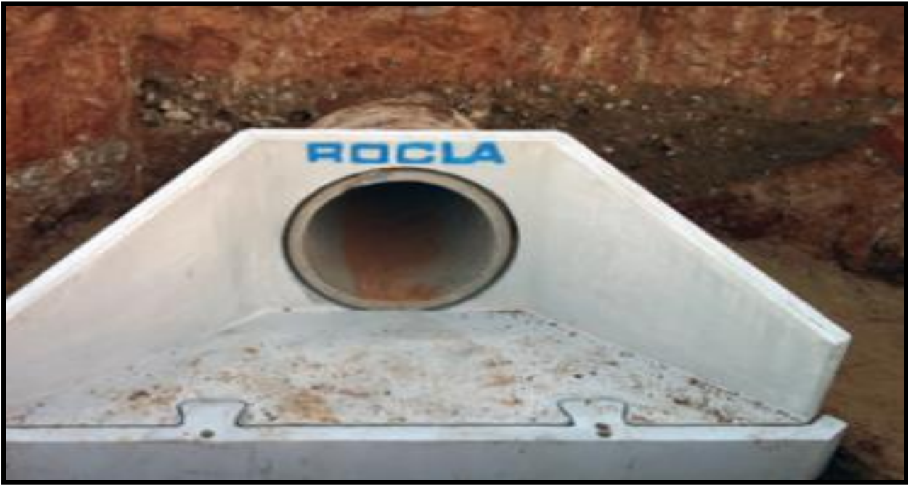
Figure 1: Showing a precast concrete pipe culvert with concrete headwalls
