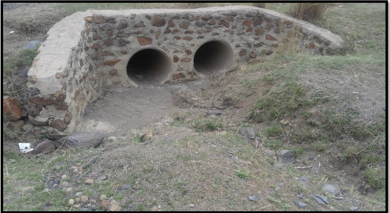
Figure 2: Showing concrete pipe culvert with stone pitched headwalls.
