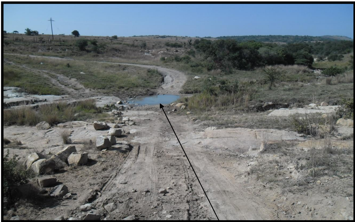
Photo 3: showing existing road and proposed causeway construction.
