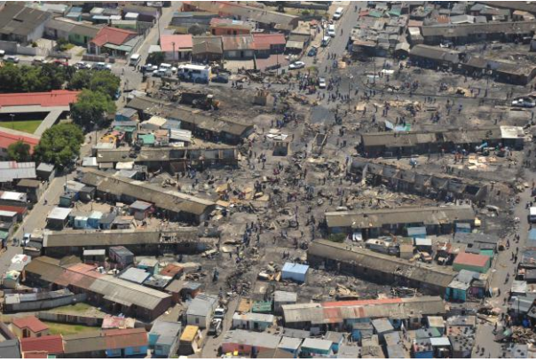
Aerial View of Langa Hostels after the fire in March 2012, CCT 2011
