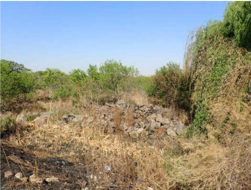
Figure 31 Dumped dolomite rock within the original drainage feature
