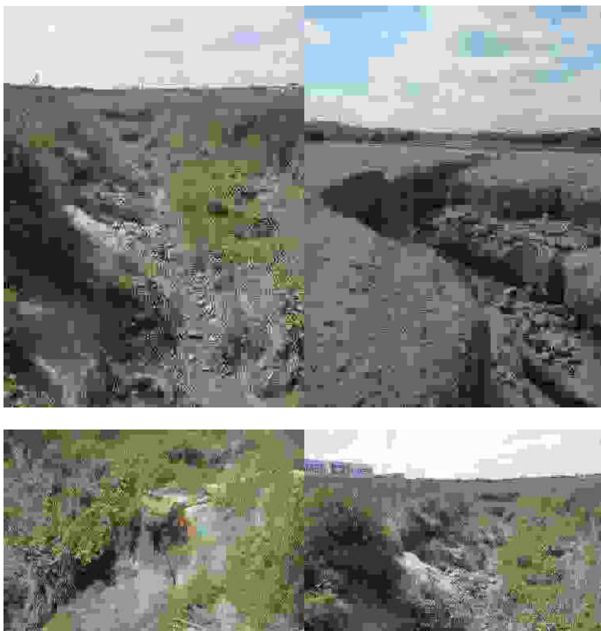
Figure 3: Photographs indicating severe erosion and degradation in the watercourse prior to rehabilitation.
