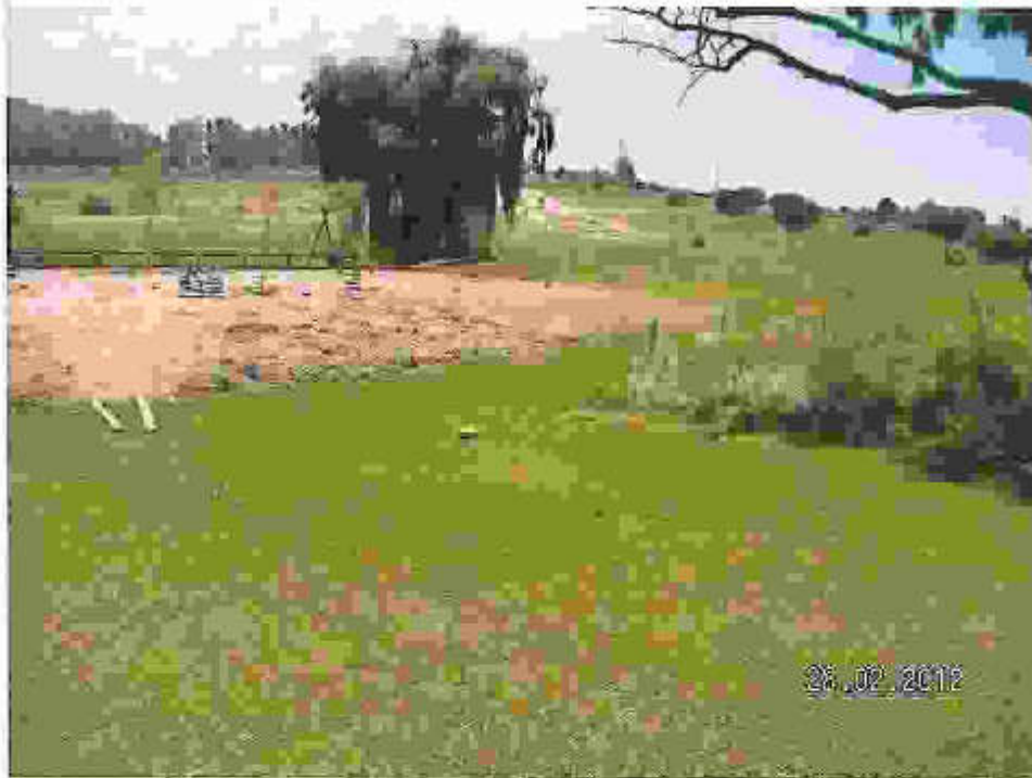
Figure 8: A play area was constructed within a sensitive wetland area
