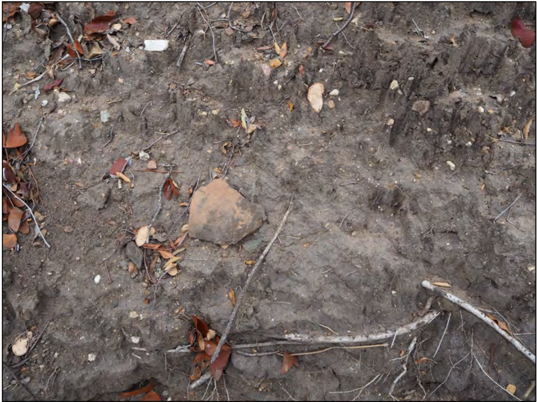
Figure 22. Deposits within vertical erosion wall
