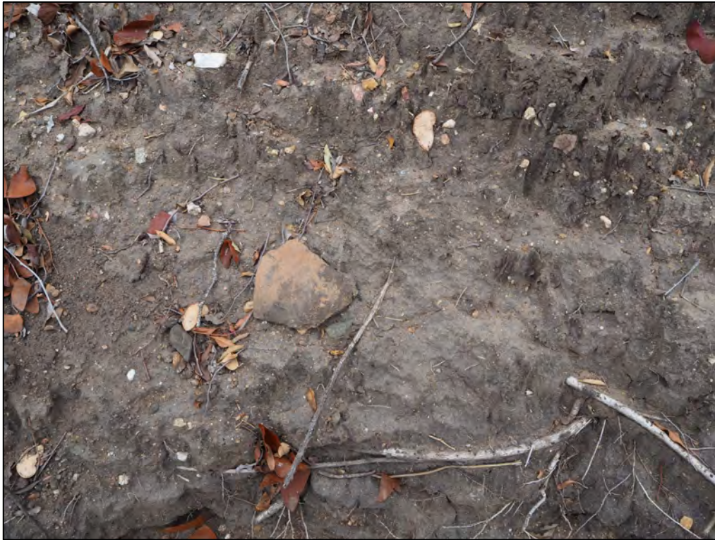
Figure 27. Exposed wall at Site 1
