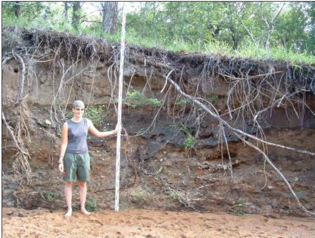
Figure 28. Eroded wall from Antonites Report (Antonites, 2005)
