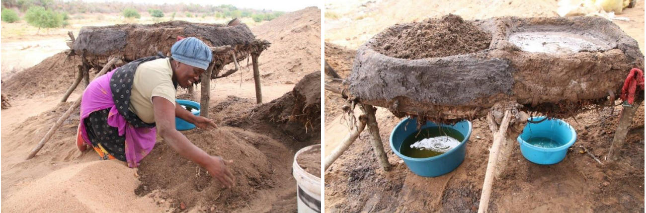
Figure 5: Soil collected from the wetland's edge is mixed with river sand before being placed in the filters.
