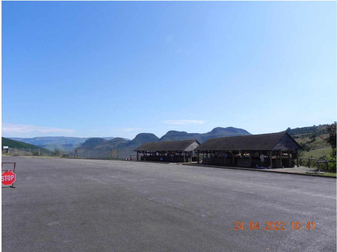
Figure 18: Lisbon Falls entrance
