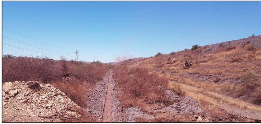
PLATE 4-2: EXISTING ASBESTOS-LINED SOLUTION TRENCH AT THE TOE OF THE TAILINGS SAMS
