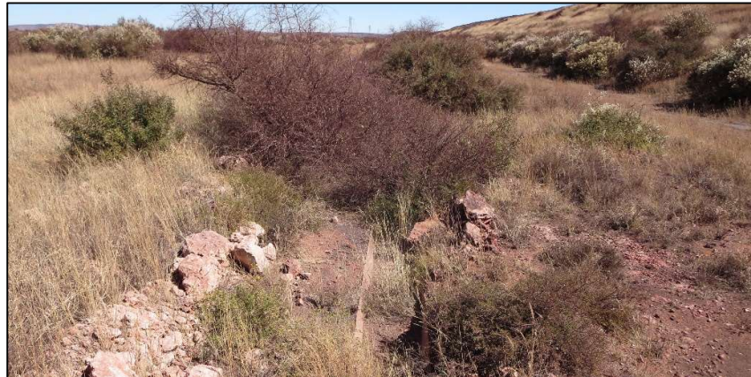
PLATE 4-3: EXISTING SOLUTION TRENCH OVERGROWN WITH VEGETATION AND FILLED WITH SEDIMENT
