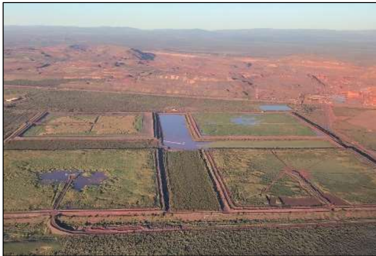
PLATE 4-1: AERIAL VIEW OF CURRENT TSF
