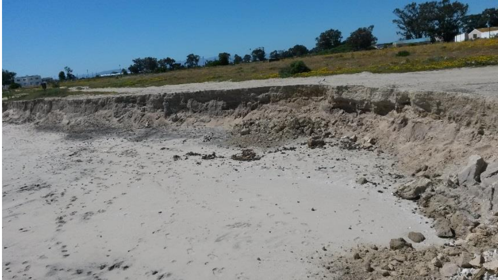
Figure 2-10 Evidence of Coastal Erosion on the Hangbos Side of the Harbour
