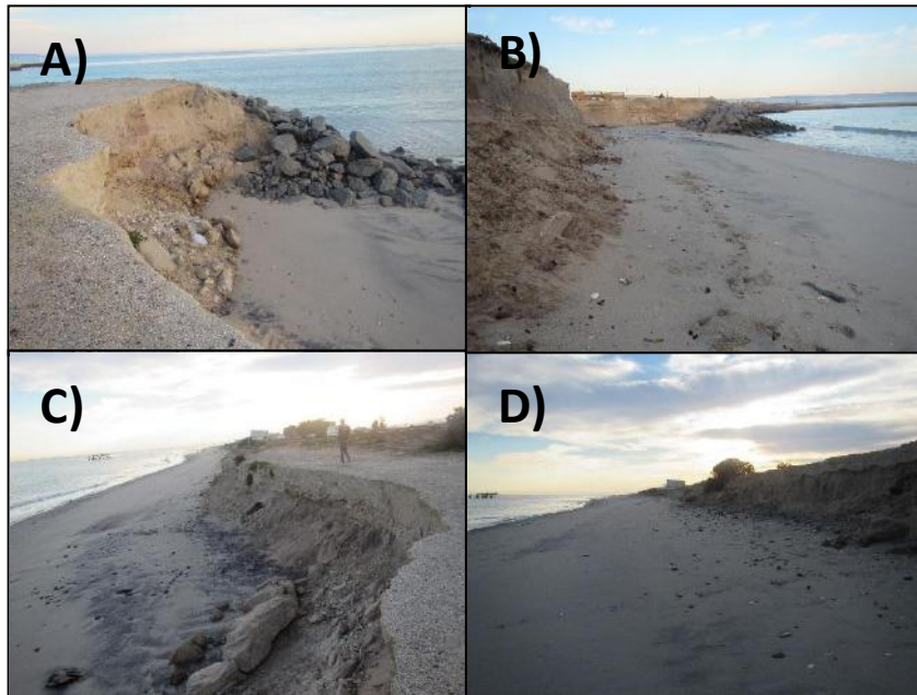
Figure 2-1: Photos taken of the sediment receiving beach (north east of the harbour) just after spring low tide (8 am) on the 23rd May 2017. A) View from the top of the eroded cliffs towards the shore armouring; B) View from site LH 5 looking south west towards the harbour; C & D) Two views of the steeply sloping beach profile, alongshore towards the north east.
