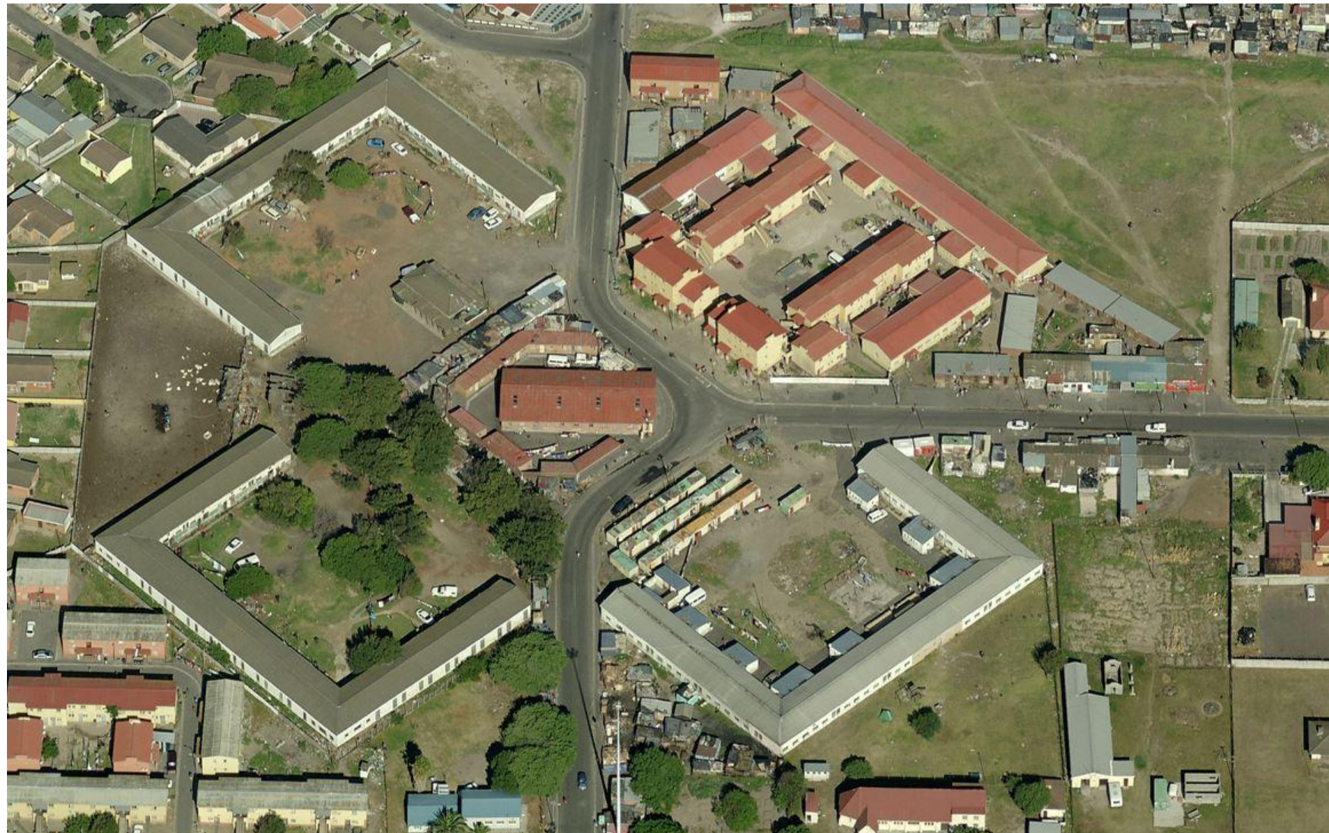
Oblique aerial view of the Main Barracks, facing eastward
