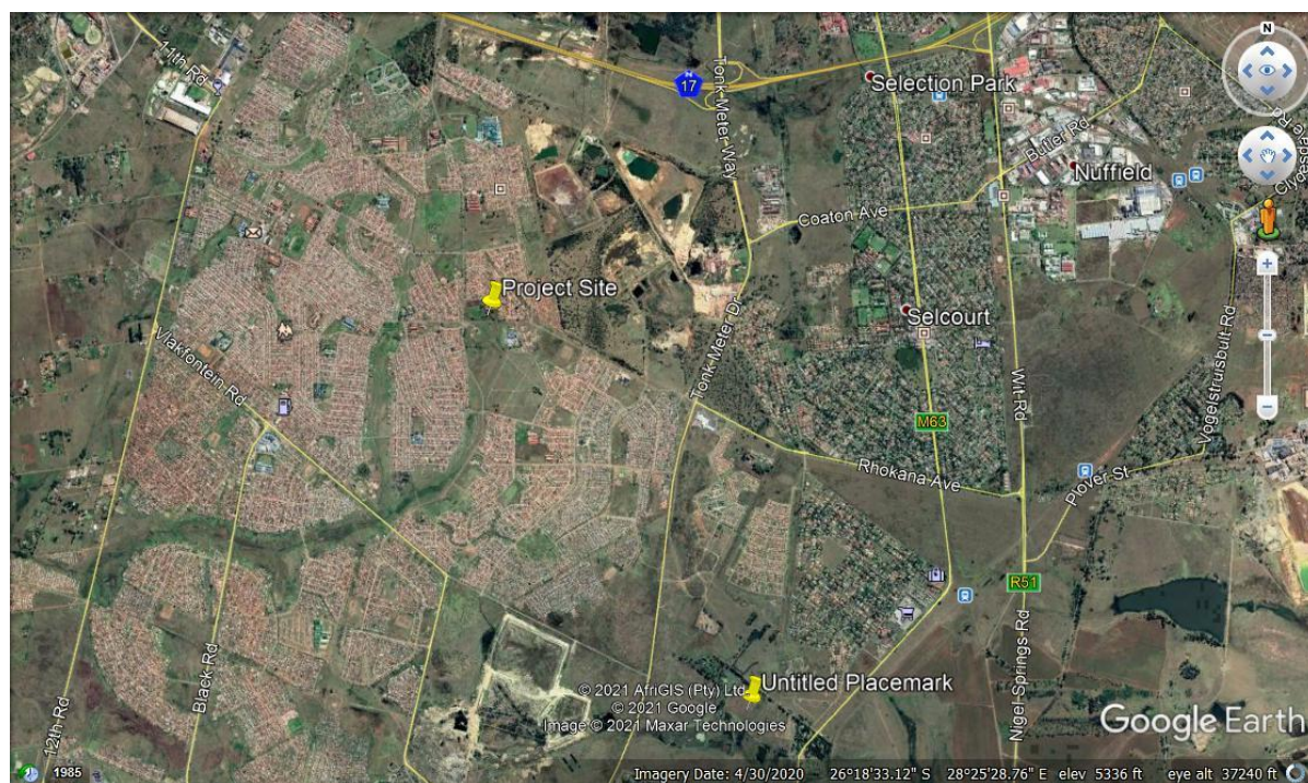
Figure 2: Overview of already existing access roads to site
