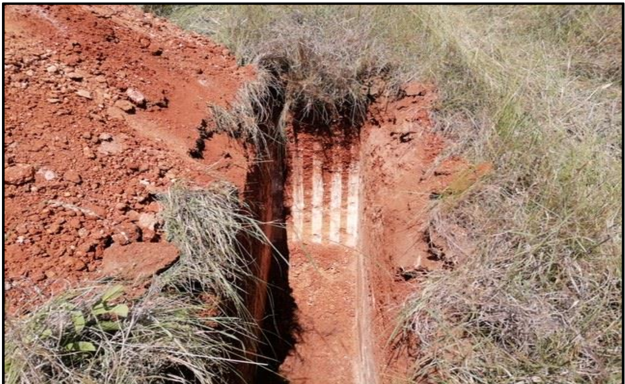
Figure 2: A photograph showing a typical trial pit on site
