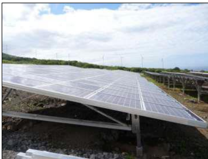
FIGURE 3: FIXED SOLAR PV PANELS.
