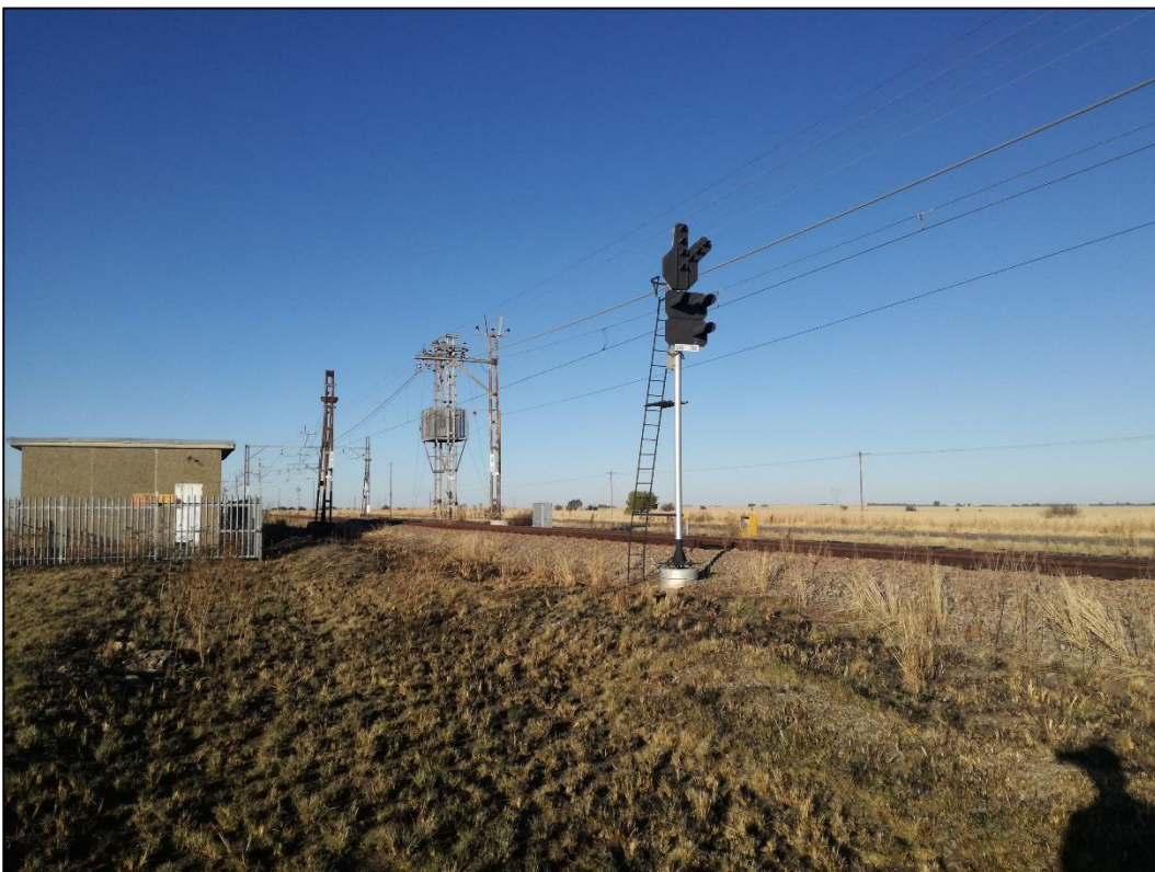
Figure 15: Railway infrastructure adjacent to the R502 Main Road
