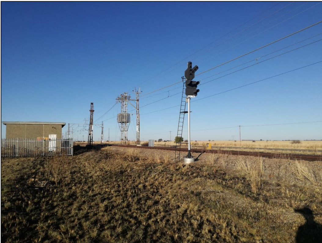
Figure 16: Railway infrastructure adjacent to the R502 Main Road
