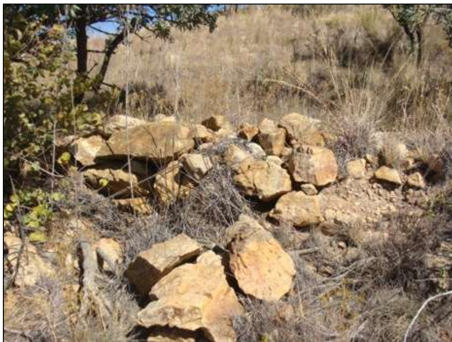
Photo 5: Military stone walling at site no. 5.
