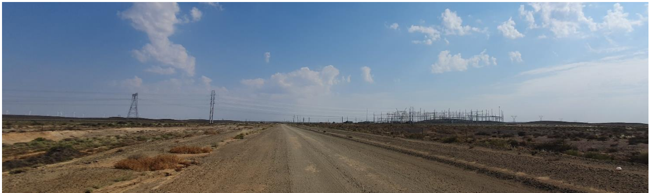
Figure 5-3: Existing network of powerlines converging at the Helios MTS. Photograph is taken looking north.
